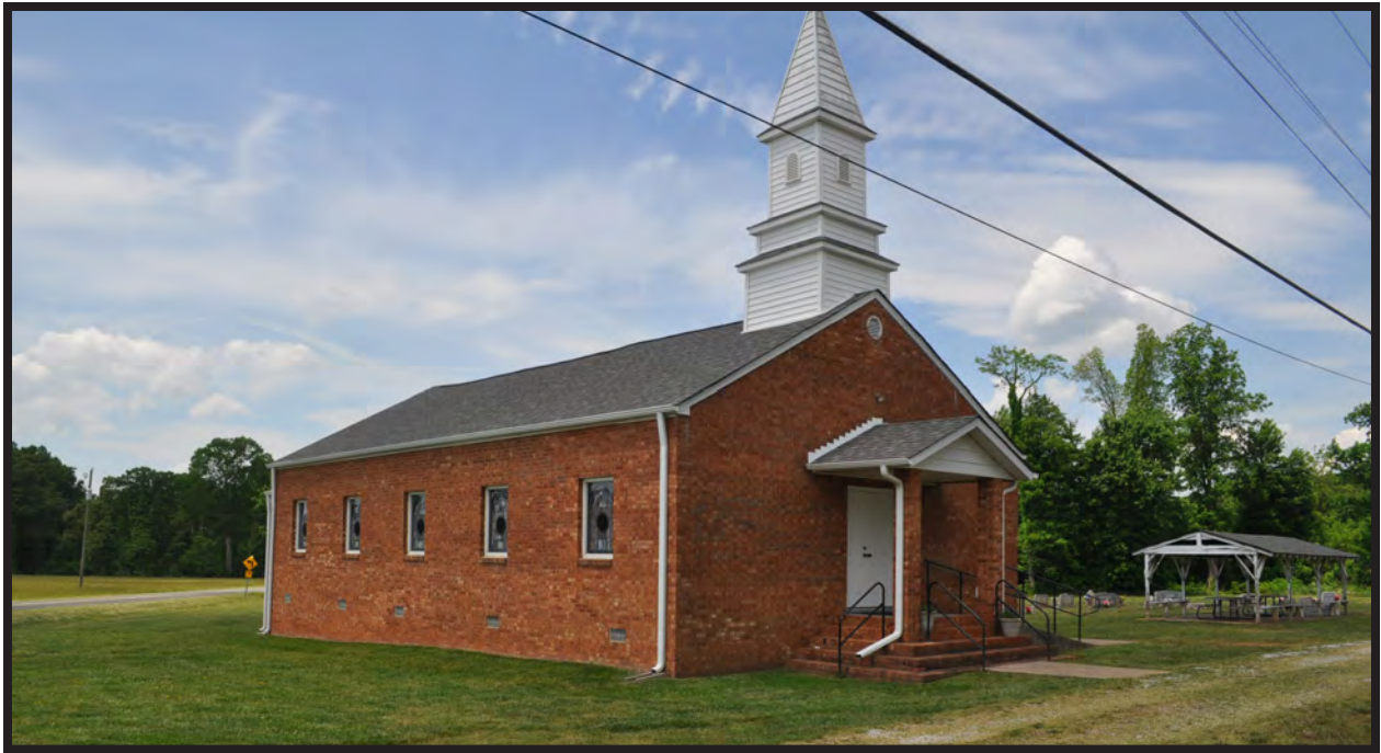
Figure 5. Front (Northeast) and Southeast Sides
