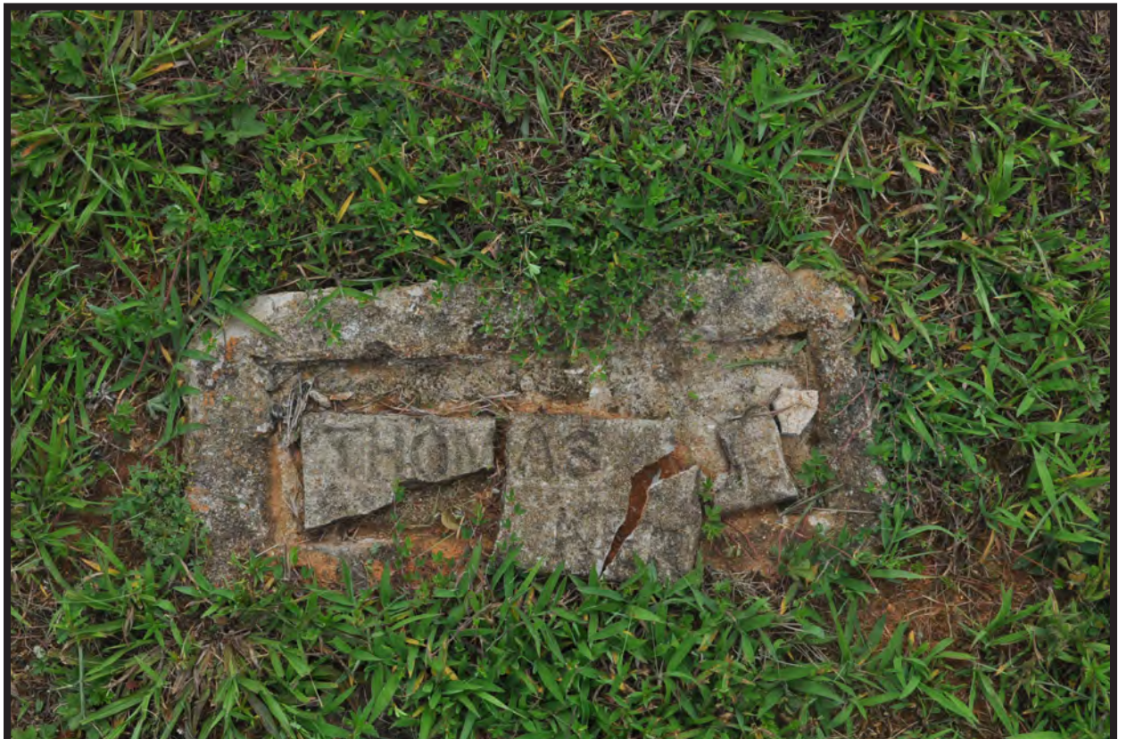
Figure 18. Concrete Marker with Broken Name Plate
