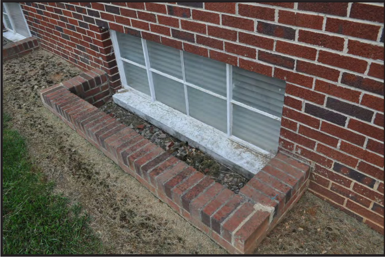
Figure 28. Basement Window Well
