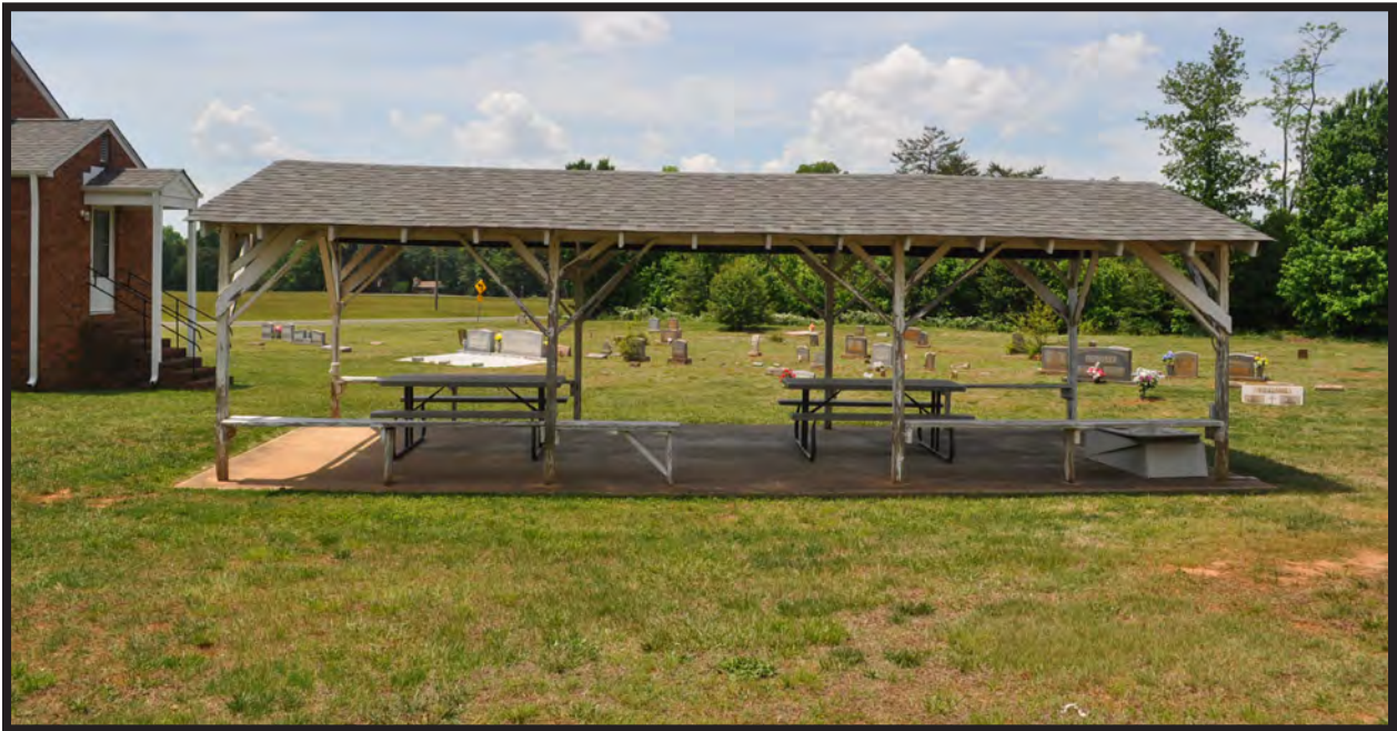
Figure 12. Picnic Shelter, Looking West
